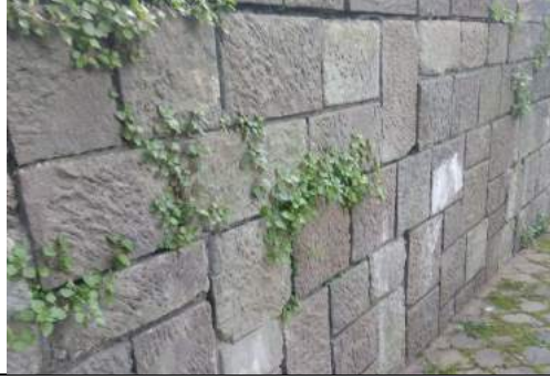
Architectural Reality: KTU library garden wall
