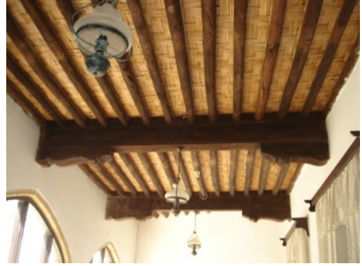
Figure 7. Ceiling with wooden main beams (By Author)
